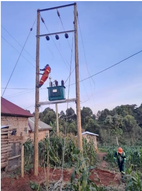
Figure 13: Construction of 3-phase electric power at for the facility in Mityana
