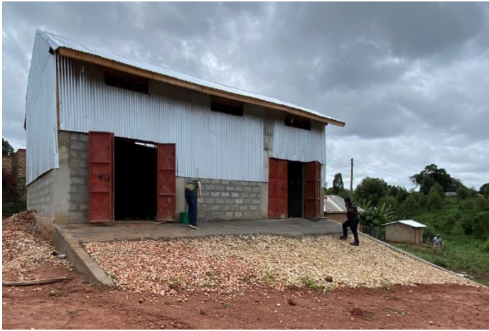
Figure 12: Processing facility in Mityana
